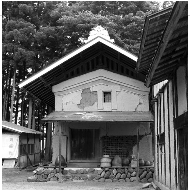
A three-hundred-year-old storehouse ( kura ) with walls damaged in an earthquake.
